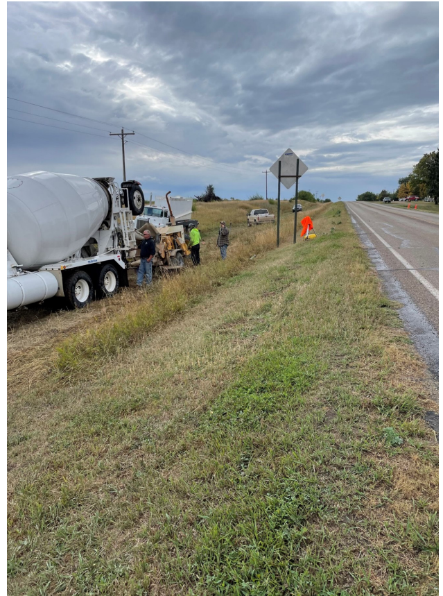
Pumping Grout Near Highway 15 in Garrison
