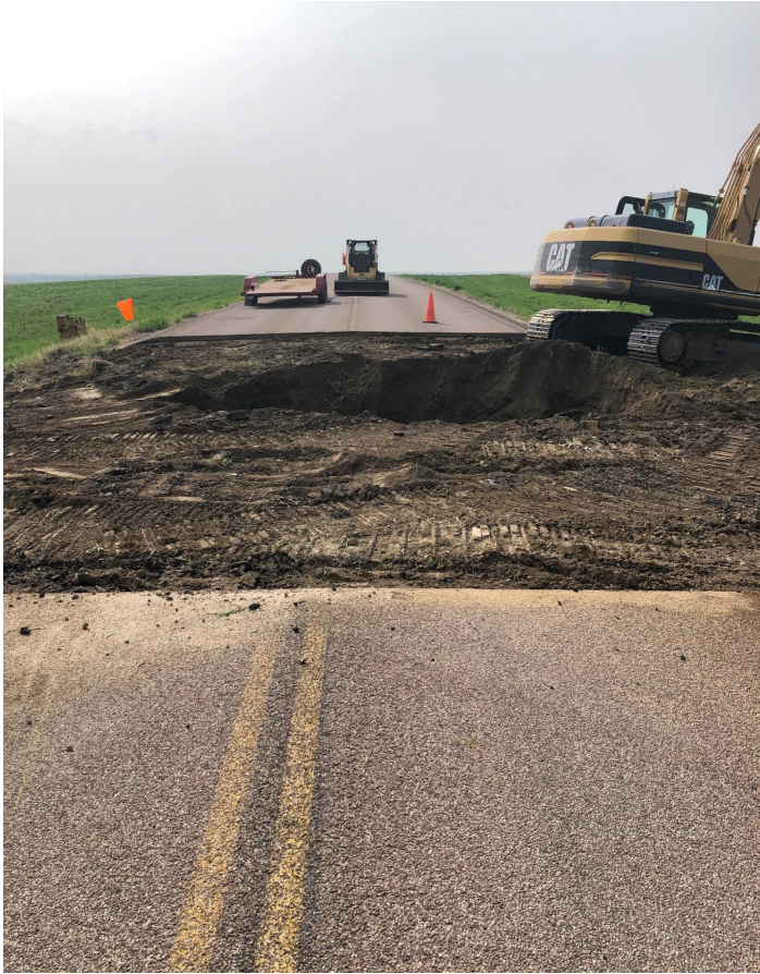
Excavator Digs up Sinkhole that Formed Under Highway 12 Near Scranton
